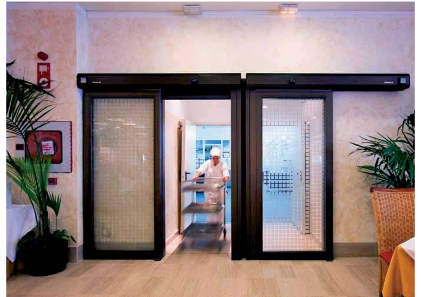
Fire-resistant door separating kitchen and restaurant. Hotel sector.
