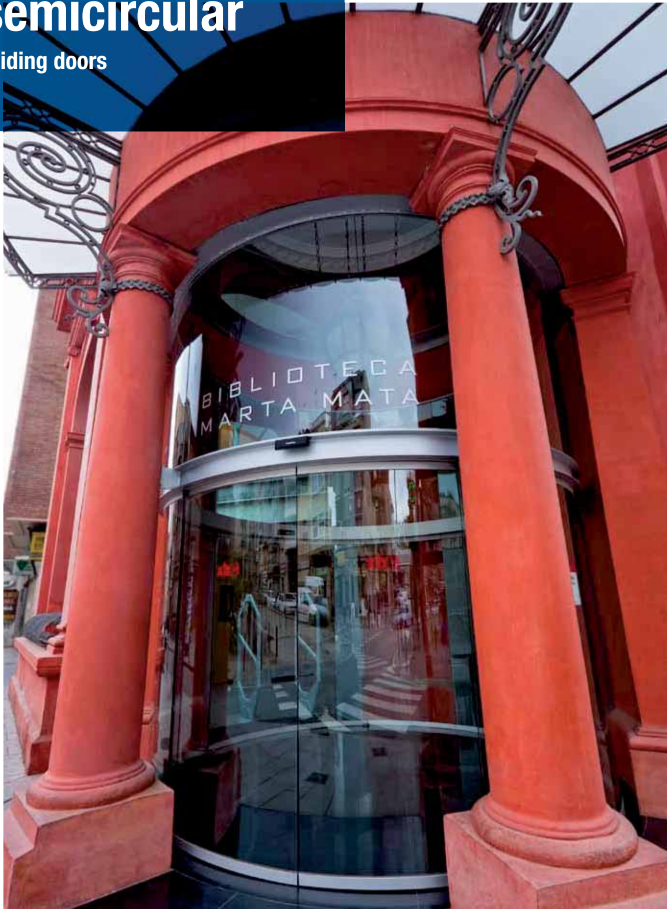
Circular automatic door. Library.
