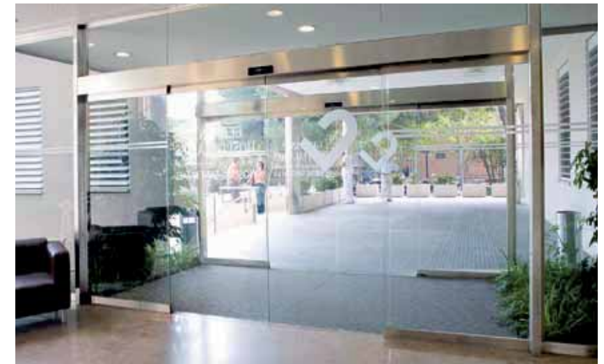
Entrance with two bi-parting sliding doors. Hospital.
